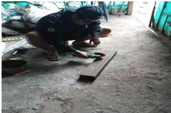
Figure 2. U . Channel Iron Cutting
